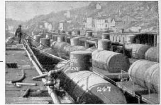
BOILER TANK CARS
